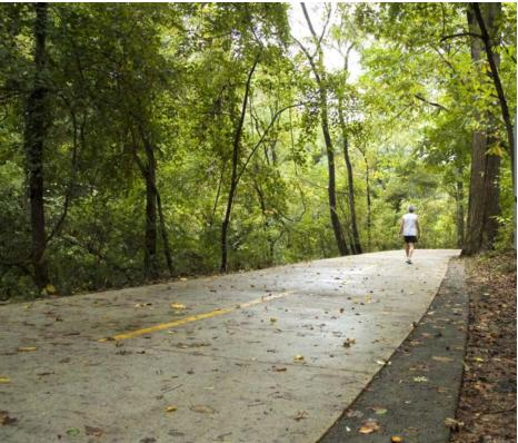
Tree root bridging allows the trail to come close to specimen trees without causing harm while a porous concrete edge aids infiltration.
