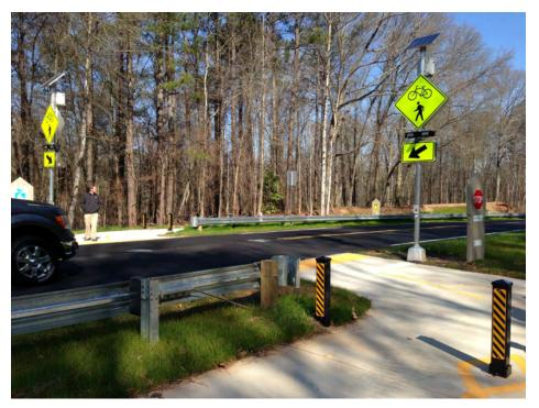
Example of crossing with a rapid flashing beacon.
