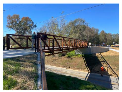
Prefabricated bridge on the Firefly Trail in Greene County.
